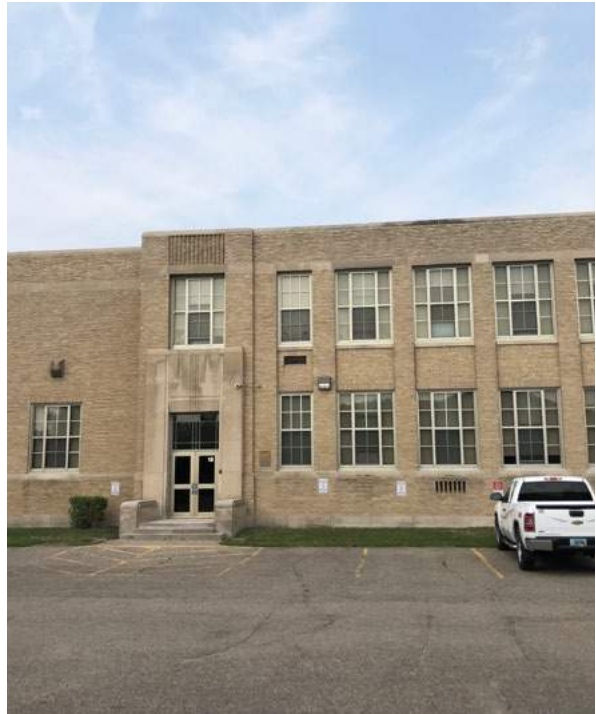
Exterior entrances are missing adequate handrails and guardrails, and do not have required ramps or handicap accessible entrances.
