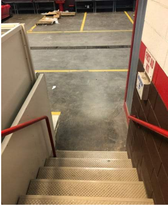
Hand and guard rails are not handicap accessible in automotive technology and construction trades classrooms.
