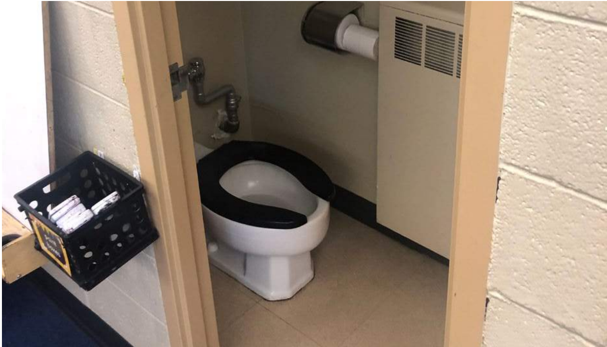
Restrooms within classrooms are very small and do not meet maneuverability and clearance requirements.
