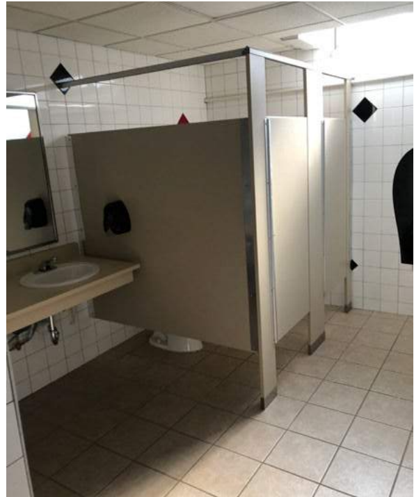
No handicap accessible toilet or sink in women's locker room.
