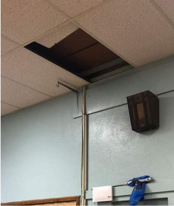
Missing ceiling tiles, and exposed wiring throughout the school.
