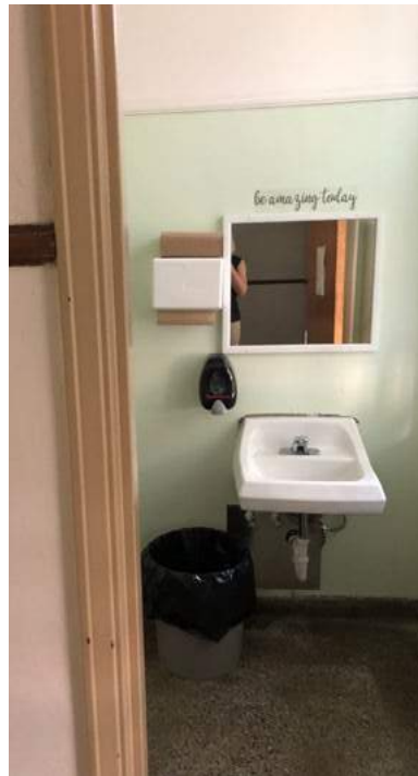
Staff restrooms are not handicap accessible. Stalls are not ADA compliant, sinks are not accessible.
