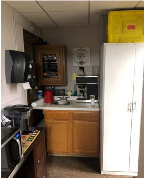
Break room in main office is not handicap accessible. Sink is too small, too high, and too far back. Space does not meet maneuverability clearance requirements.
