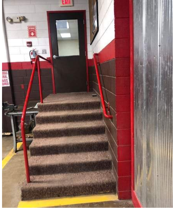
Hand and guard rails are not handicap accessible in automotive technology and construction trades classrooms.
