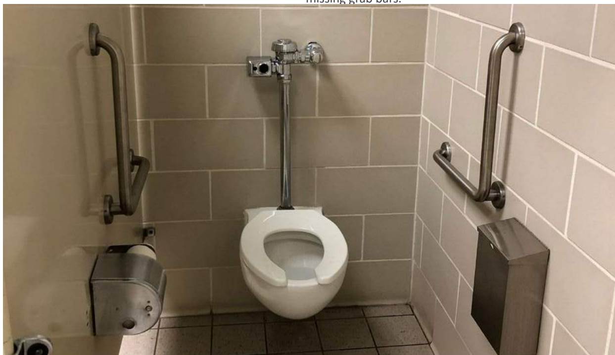
Grab bars in ADA stalls are not all code compliant in men's and women's restrooms.
