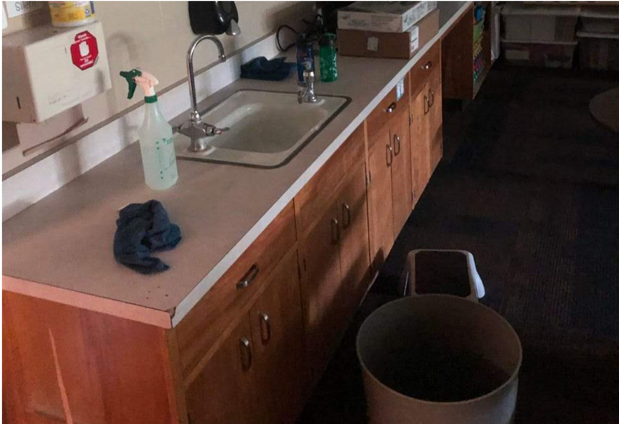
Sink has drinking fountain bubbler on it, which is not up to code and does not meet handicap accessibility clearances.
