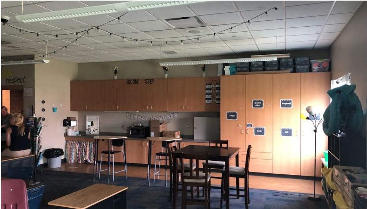
Sink in new casework is not handicap accessible because of exposed plumbing underneath.
