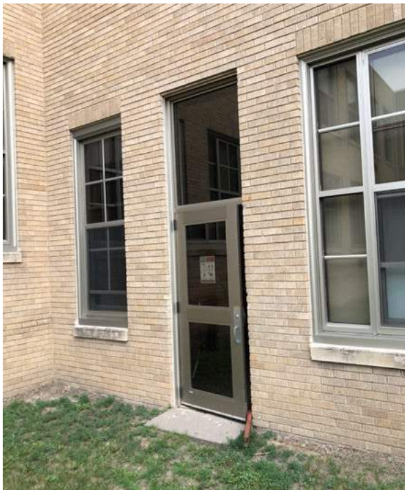
No accessible entrance to the courtyard and no exit out of the courtyard.
