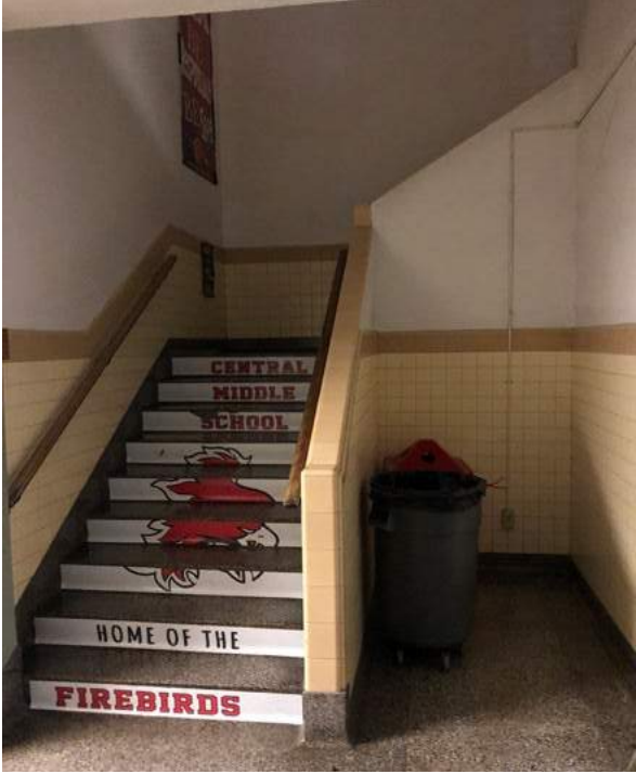
Staircases are not enclosed and do not lead directly to exterior. Handrail and guardrails are missing or not code compliant.
