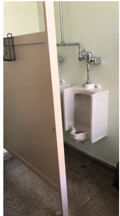
Staff restrooms are not handicap accessible. Stalls are not ADA compliant, sinks are not accessible.
