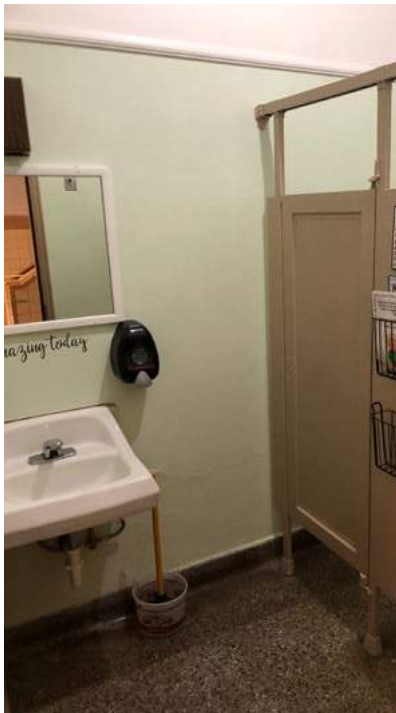
Staff restrooms are not handicap accessible. Stalls are not ADA compliant, sinks are not accessible.
