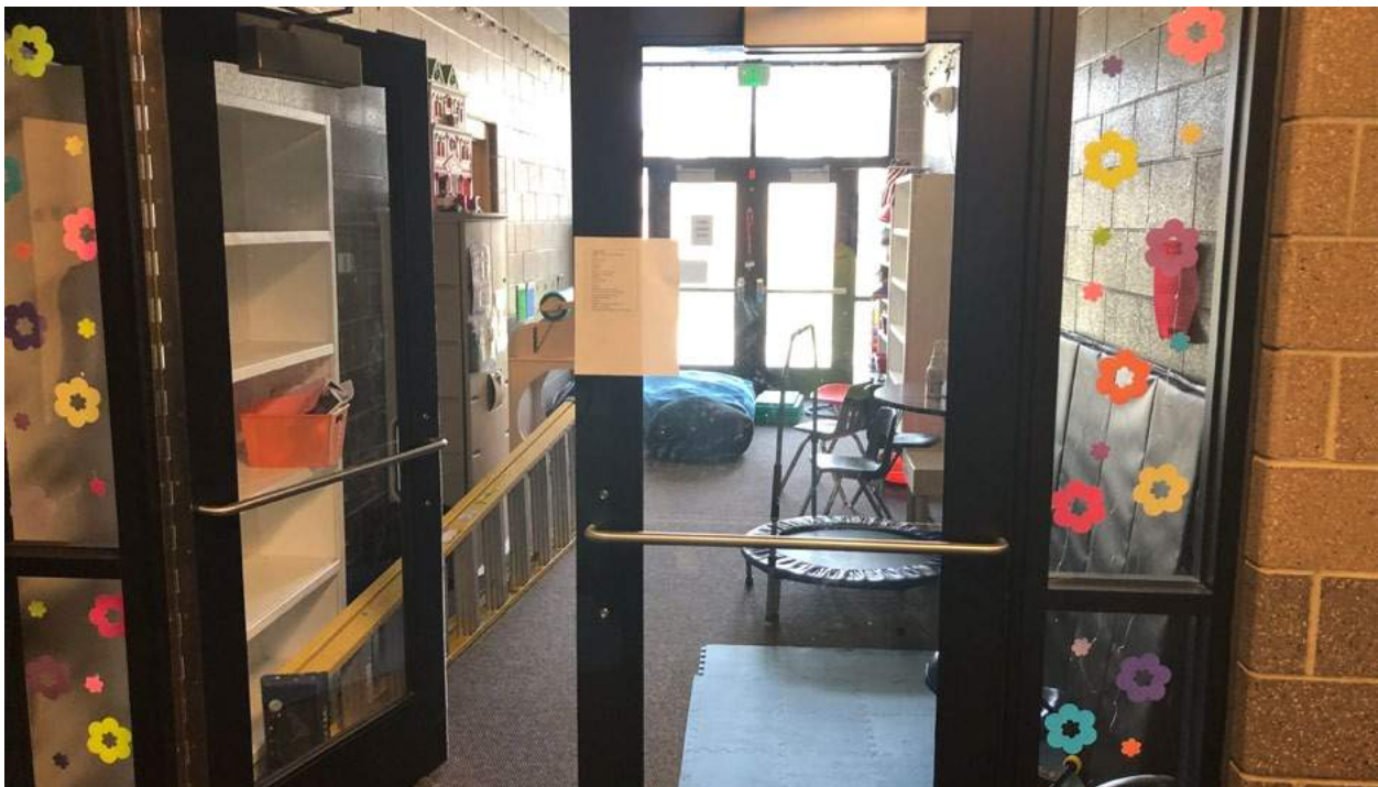
Exit vestibule used as a classroom space, does not meet fire code.
