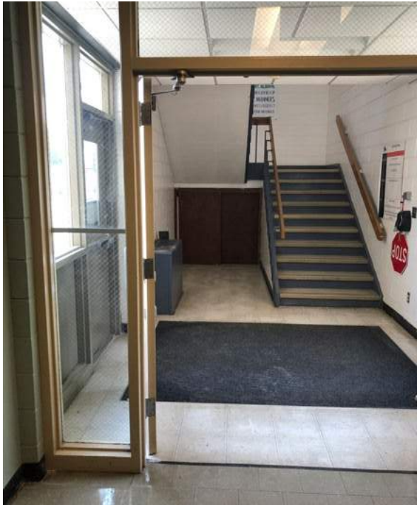
Door 10 has wire in the vestibule windows, this is no longer to code.
