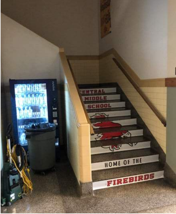
Staircases are not enclosed and do not lead directly to exterior. Handrail and guardrails are missing or not code compliant.
