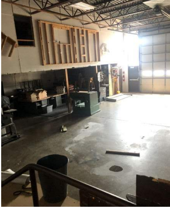
Mezzanine in construction technology area is not handicap accessible and is not to code because it is enclosed.
