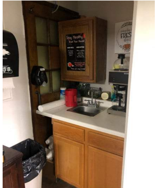
Break room in main office is not handicap accessible. Sink is too small, too high, and too far back. Space does not meet maneuverability clearance requirements.
