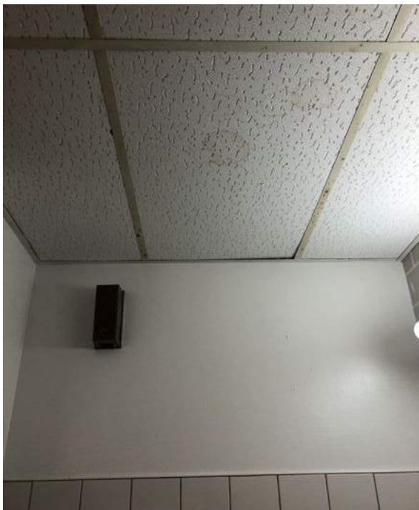
Ceiling tile in bad shape and has water damage in bathrooms.
