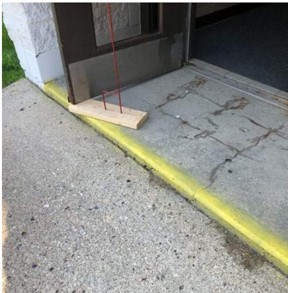
Sidewalk outside of Door 3 has sunk and is no longer handicap accessible.
