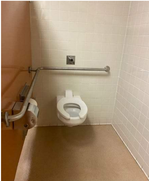
The ADA stall is not handicap accessible in the women's restroom due to grab bars, vertical bar, and stall width. The sinks in the women's restroom are not handicap accessible.
