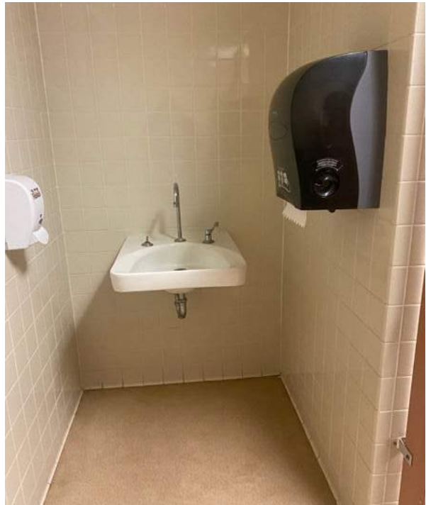
The ADA stall is not handicap accessible in the women's restroom due to grab bars, vertical bar, and stall width. The sinks in the women's restroom are not handicap accessible.
