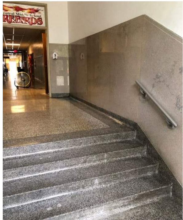
Door 2: Handrails are not to code. No middle railing. Not an accessible entrance.
