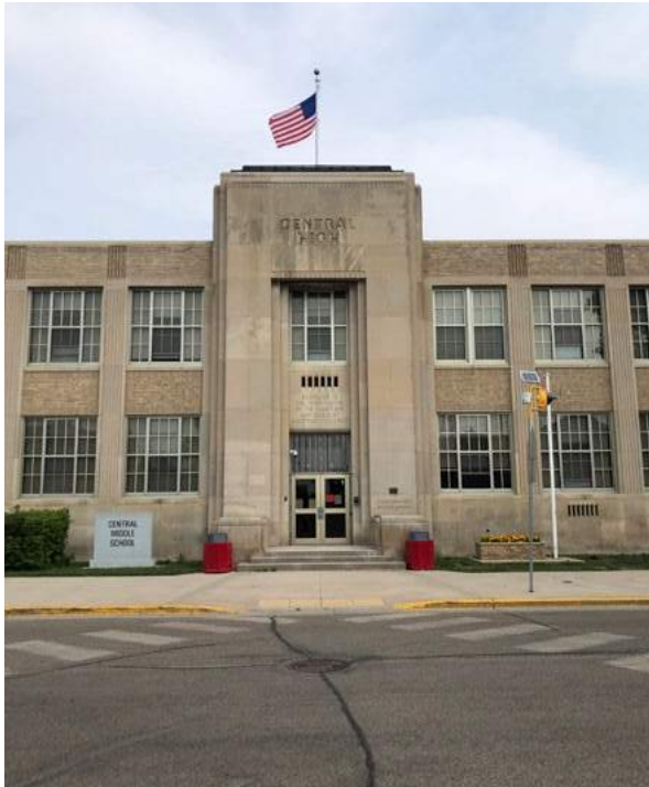
Exterior entrances are missing adequate handrails and guardrails, and do not have required ramps or handicap accessible entrances.
