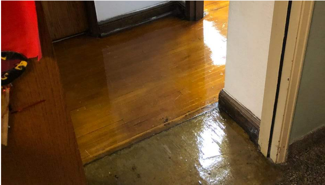
Classroom entrances are not wide enough for maneuverability clearances for ADA compliance.
