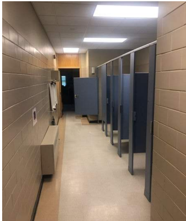
Restrooms within classrooms are very small and do not meet maneuverability and clearance requirements.
